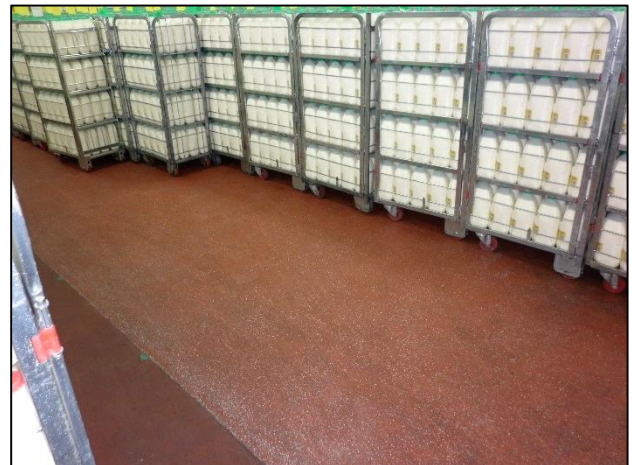
Examples of good floor surfaces on which a maximum of two trolleys could be moved, subject to risk assessment
