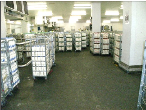
Examples of good floor surfaces on which a maximum of two trolleys could be moved, subject to risk assessment
