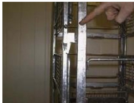
Missing or damaged latch / catches
